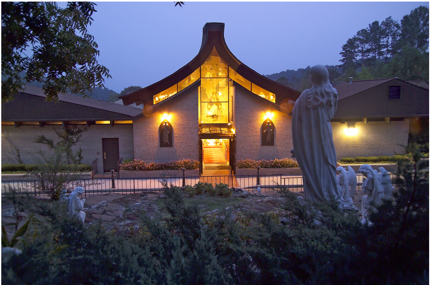
The chapel on the grounds of the EWTN offices and studio in Irondale, Alabama. (Courtesy of EWTN)
