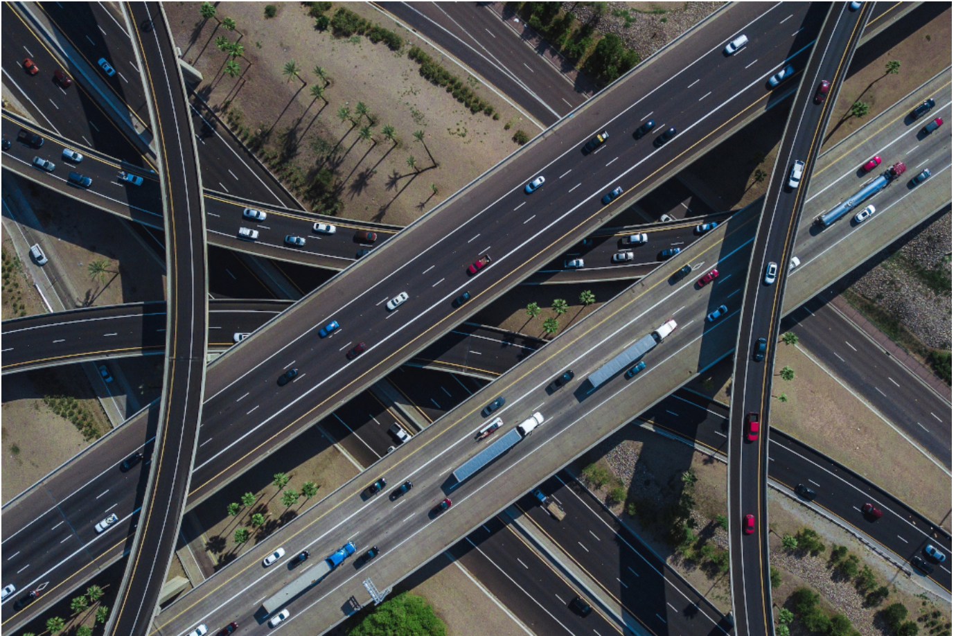
Vehicles travel along multiple layers of overpasses in Phoenix, Arizona. (Unsplash/Creative Commons/Jared Murray)
