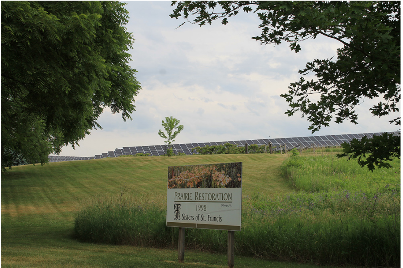
An array of 2,600 solar panels in the background of a restored prairie area at the motherhouse of the Sisters of St. Francis, in Dubuque, Iowa. (EarthBeat photo/Brian Roewe)
