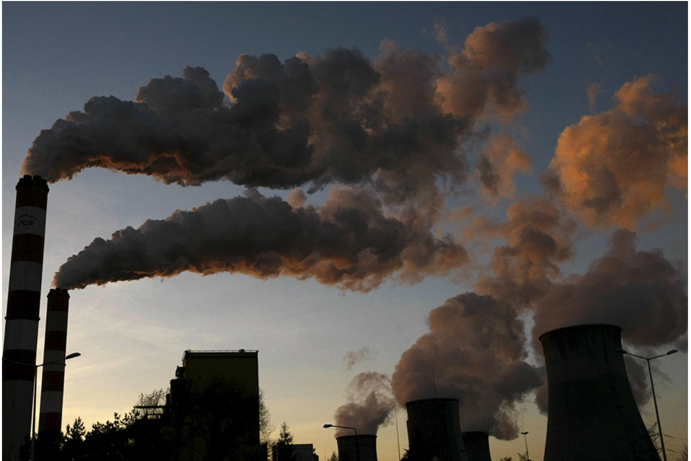
Smoke billows from the chimneys of power plant in 2014 in Belchatow, Poland. (CNS/Reuters/Kacper Pempel)
