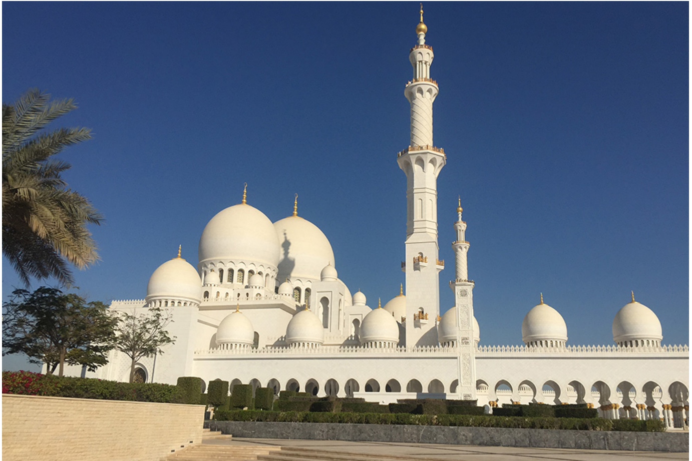
The Sheikh Zayed Grand Mosque, in Abu Dhabi, United Arab Emirates (Courtesy of Tom Gallagher)
