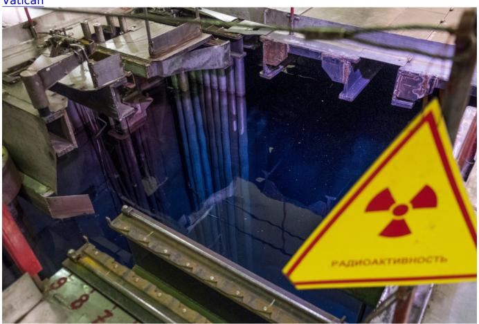
Fuel assemblies are pictured in water with a sign reading "Radioactivity" at a wet spent fuel storage facility in Chernobyl, Ukraine, in this handout image taken in May 2017. (CNS photo/European Bank for Reconstruction and Development/handout via Reuters)
