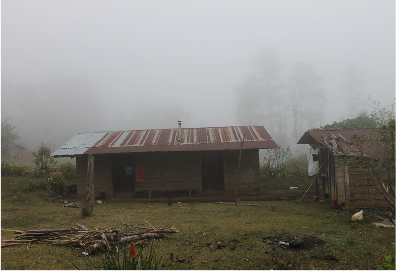
Lino Alberto's home is located in the El Cedro community of Opatoro in La Paz. Category 4 hurricanes, Eta and Iota, struck Honduras days apart in November 2020. While the hurricanes made landfall along the northeast coast, torrential rainfall carried well into the Dry Corridor. Floodwaters swamped Alberto's fields and wiped out his entire crop.(NCR photo/Brian Roewe)
