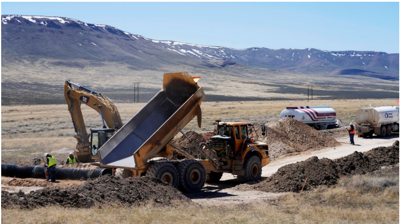
Construction continues at the Lithium Nevada Corp. mine site Thacker Pass project on April 24, 2023, near Orovada, Nev. (AP/Rick Bowmer)
