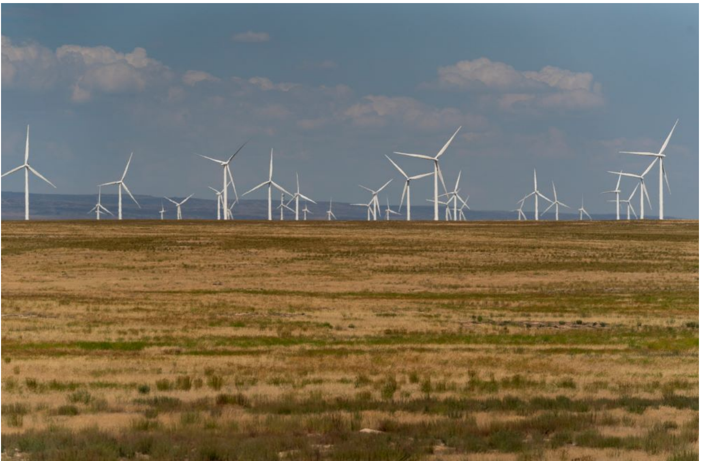
Wind turbines are seen from Interstate 84, July 9, 2023, near Hammett, Idaho. (AP/Lindsey Wasson, file)
